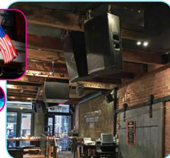
two-way speakers serving as a sidefill/delay setup to add further depth to the room's sound.
