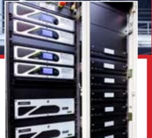
The entire system is driven by d&b's D-Series amplifiers, linked via Dante to MediaMatrix NION processing.
