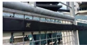
K-array's Anakonda flexible near-field/fill speakers added close-in intelligibility.
